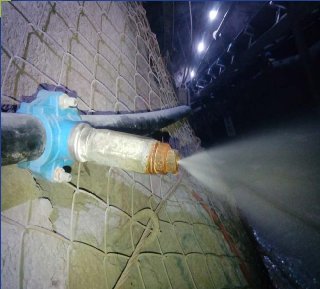
FOOTWALL TREATMENT SYSTEM IN OPERATION @ 16 BAR
